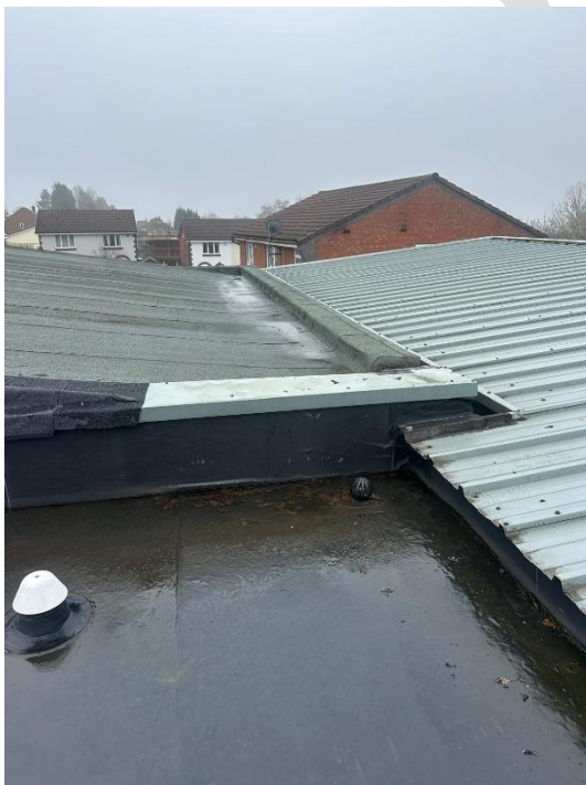
Figure 3, flat roof side overview.
